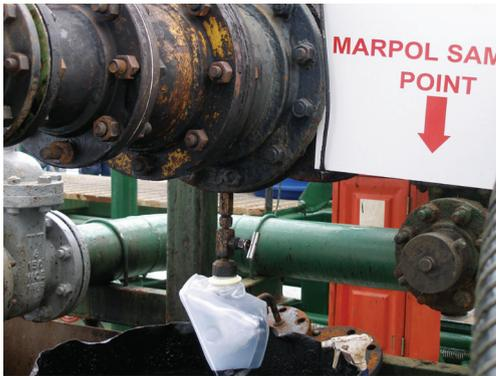
Fuel oil sampling is an essential element of any bunkering operation.
